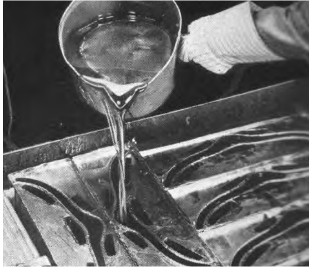
Figure 2 Production process of Catalin items: Clear syrup is poured into open leadmolds
